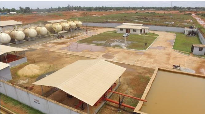
LPG-Packaging Facility by NP Liberia inside the MIP
