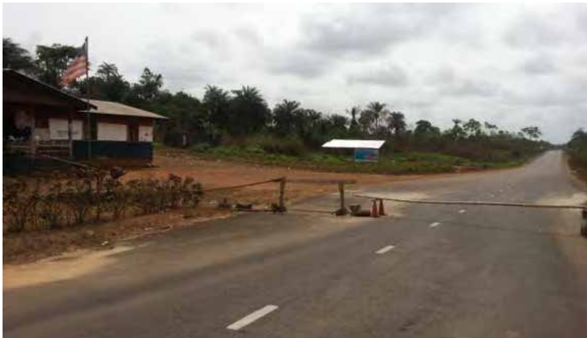
Figure III.23 Monrovia-Bo Waterside Highway Roadblock
